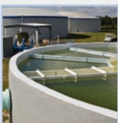
MUNICIPAL WASTEWATER TREATMENT
