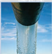
MUNICIPAL WATER TREATMENT
