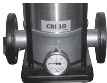
CR pump with a pressure gauge
